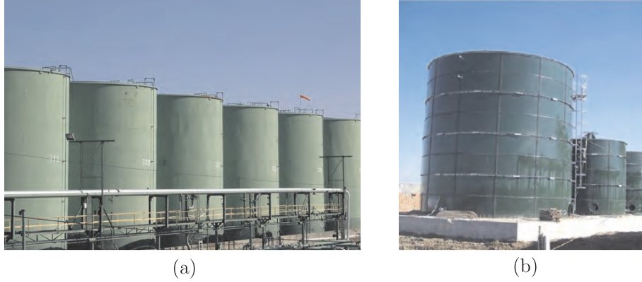
Figure 1: (a) Array of tanks in a petrochemical plant (image taken from www.joc.com , accessed on 19/01/2016); (b) cylindrical steel tanks, used to storage water, resting on a concrete foundation (image taken from www.alibaba.com , accessed on 19/01/2016).
