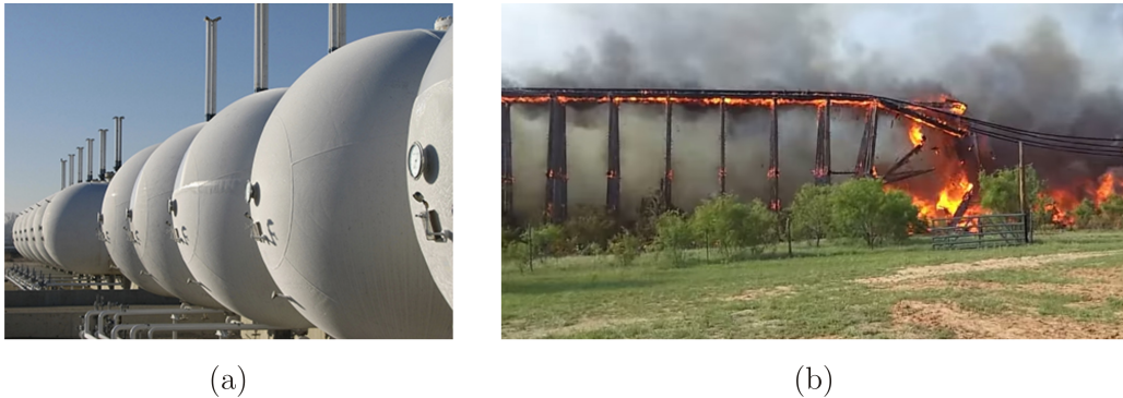
Figure 1: (a) Oil storage tanks in a power generation plant (from http://www.chromalox.com , accessed on 30 July 2015); (b) failure of the San Saba bridge in Texas, occurred in May 2013 due to fire (image captured on 30 July 2015 from the video https://www.youtube.com/watch?v=LLVKb1HxhAY ). (Online version in colour.)
